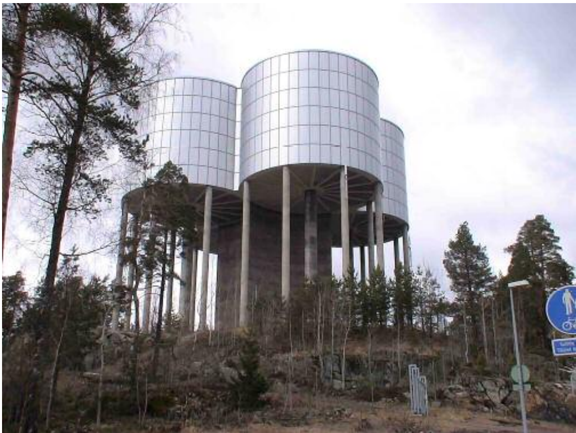
Figure 3. The Espoonlahti water tower taken into use in 1995. (Juuti 2006)
